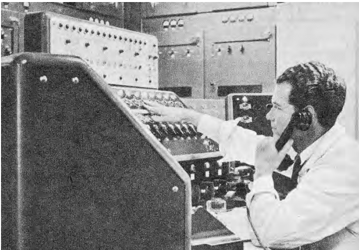
Control – “A central desk is surrounded by grey wall panels behind which are the relays”.
